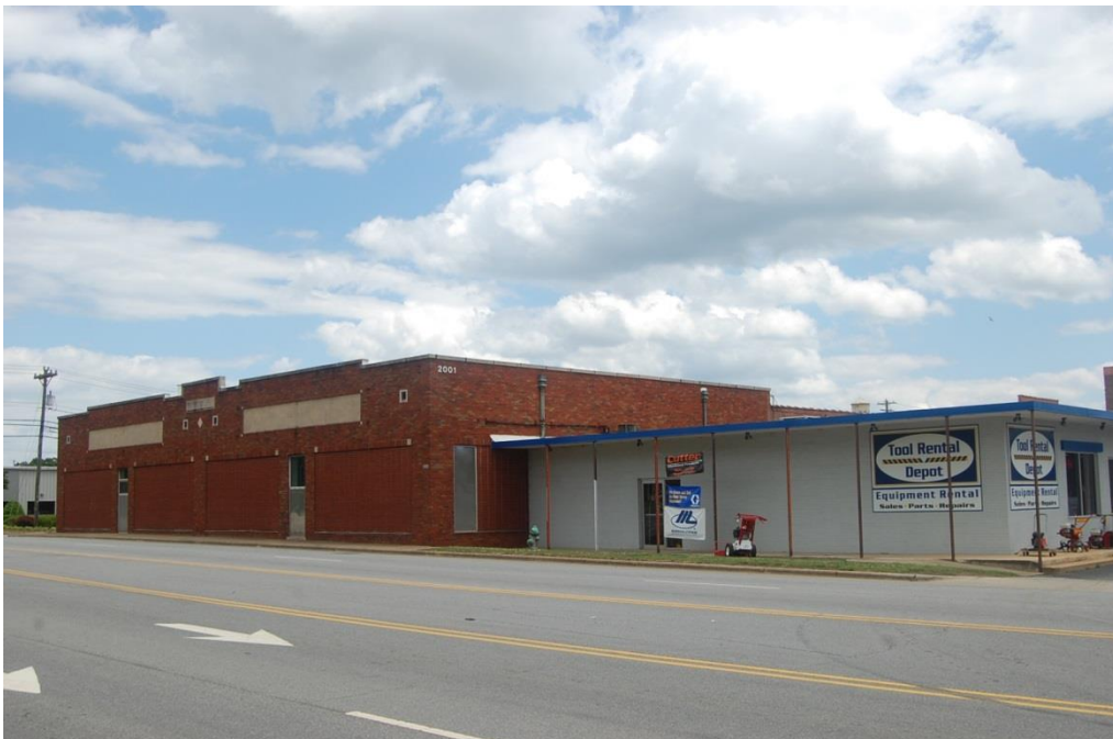
No. 25 Commercial/Industrial Building, 1929, 1953-1970s.
