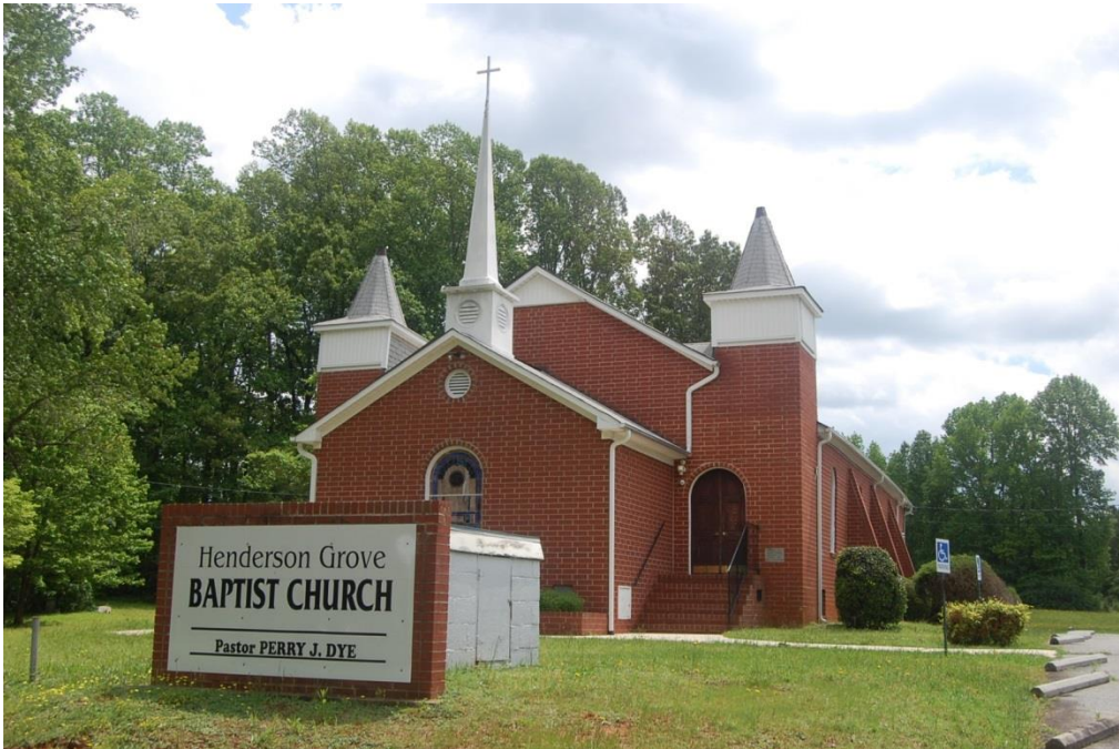
No. 1 Henderson Grove Baptist Church, circa 1912, rebuilt circa 1961
