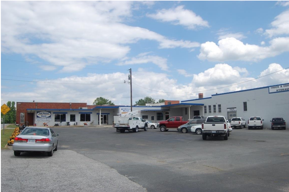
No. 25 Commercial/Industrial Building, 1953-1970s.
